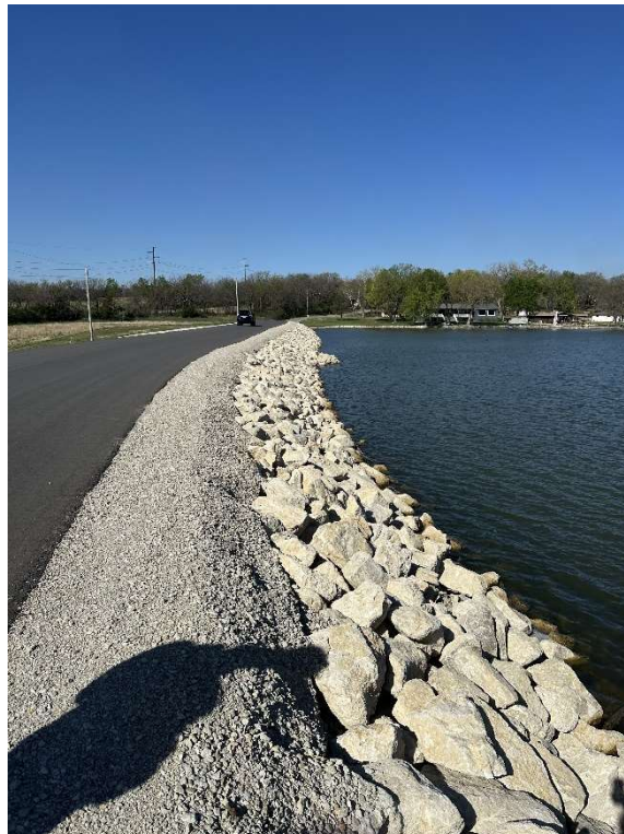
Photo #6: Standing near primary spillway looking west at upstream slope, rip rap erosion protection.
