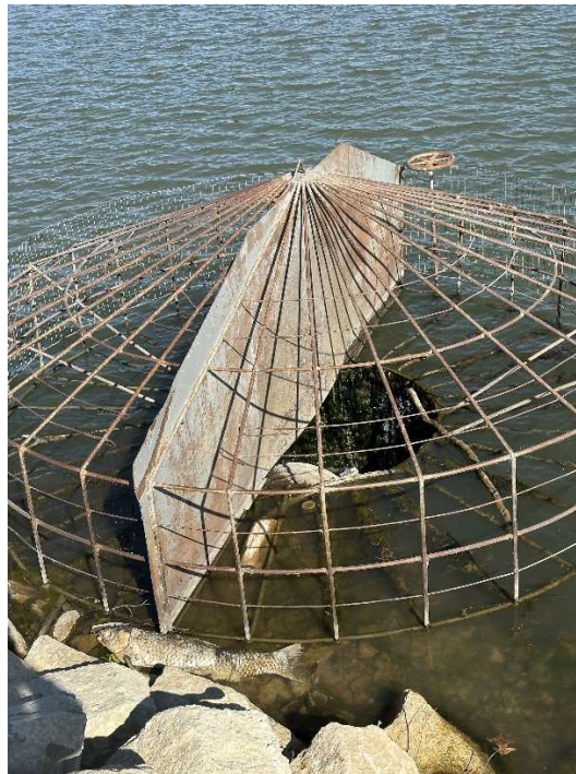
Photo #8: Primary spillway intake, CMP riser with trash rack and vortex plate.
