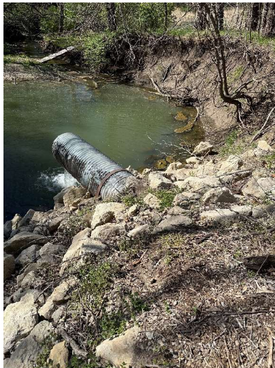
Photo #22: Primary spillway outlet.
