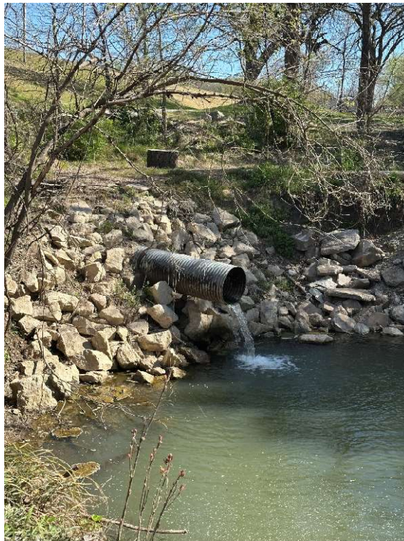
Photo #24: Primary spillway outlet.
