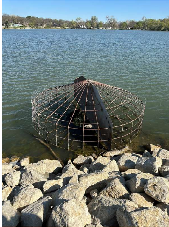
Photo #7: Primary spillway intake, CMP riser with trash rack and vortex plate.
