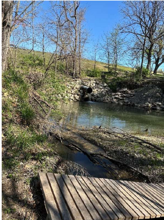
Photo #23: Primary spillway outlet.
