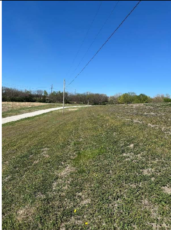
Photo #19: Power poles running along downstream slope of embankment. Power poles appear to be above the normal pool elevation.
