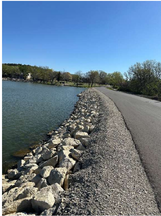
Photo #5: Standing near primary spillway looking east at the upstream slope, rip rap erosion protection.
